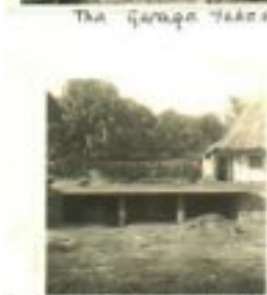
On top of garage, reinforced concrete floor of sitting-room.
