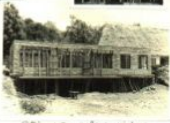
Sitting-room walls & windows.
